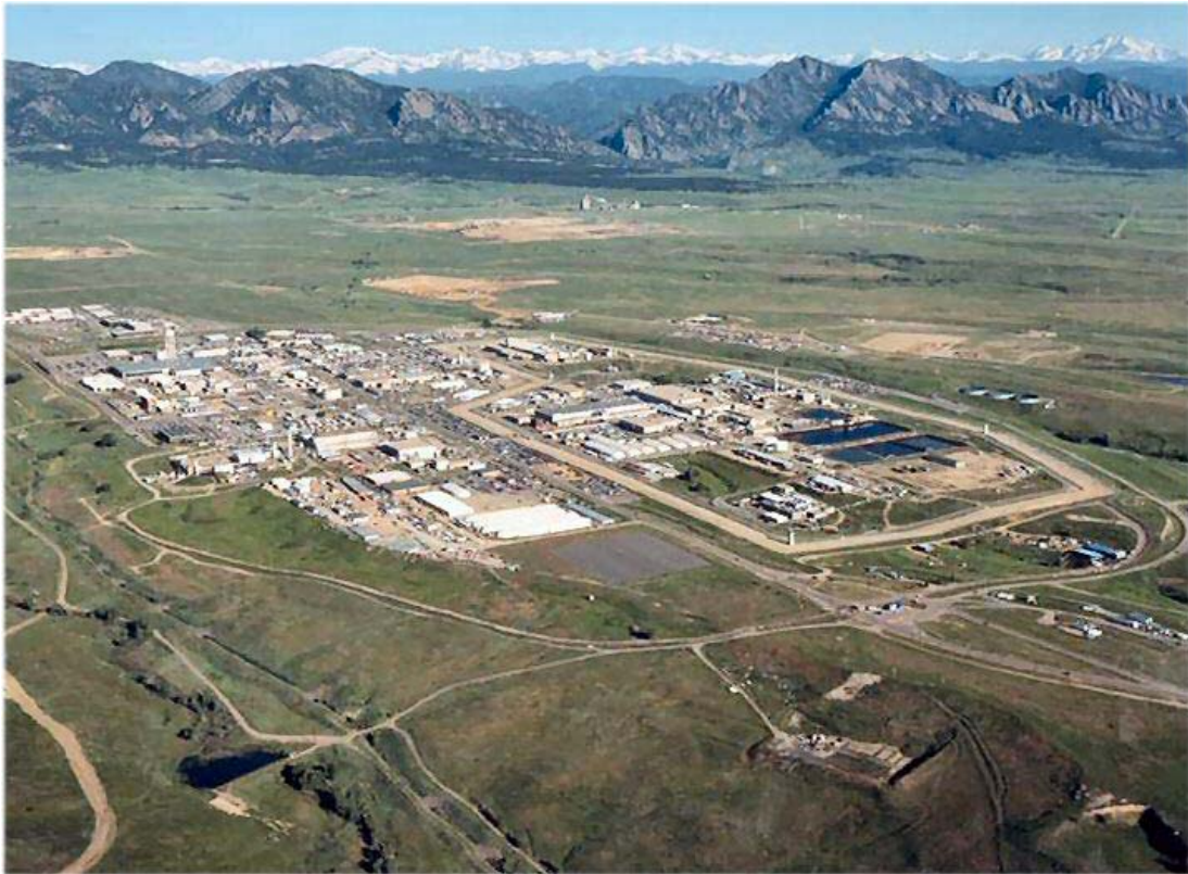
Figures 7.17. The Rocky Flats site at the height of production. What appears to be a road surrounding a portion of the industrial area is actually a high security barrier, to protect the “hot” side of the plant, where plutonium pits were produced. The other “cold” side is where non-nuclear parts made with beryllium and stainless steel were produced. Photo courtesy DOE.
