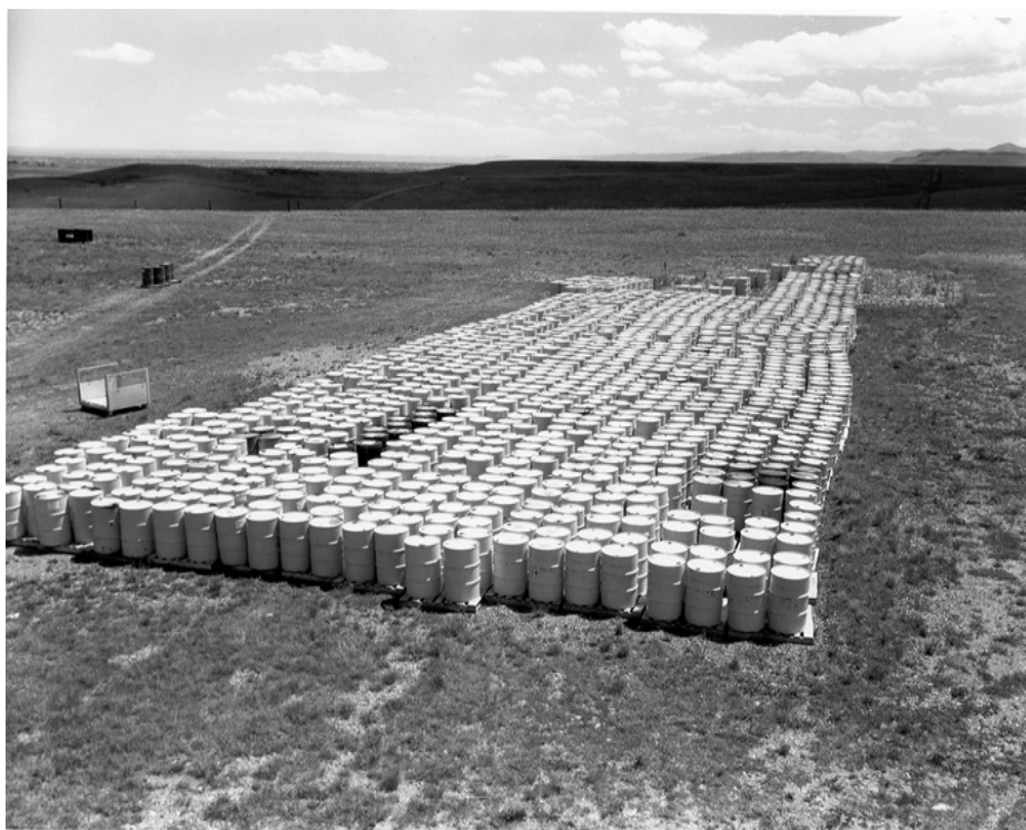
Figure 4.10: Drums of plutonium-laden waste were stored outdoors in the 903 area from 1954 until 1968. Some corroded and leaked. This area was a principal source of plutonium particles released off-site to the east and southeast. After the drums were removed, the storage area of about 260,000 square feet – bigger than four football fields – was paved with asphalt and named the “903 Pad.”
