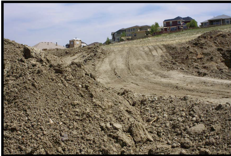
Figure 8.8: This picture of the Whisper Creek development across Indiana St. immediately SE of the Rocky Flats site dates from June 2011, when construction of houses was underway. Whisper Creek is in an area shown by Krey and Hardy in 1970 to be highly contaminated with plutonium. Photo by Robert Del Tredici.
